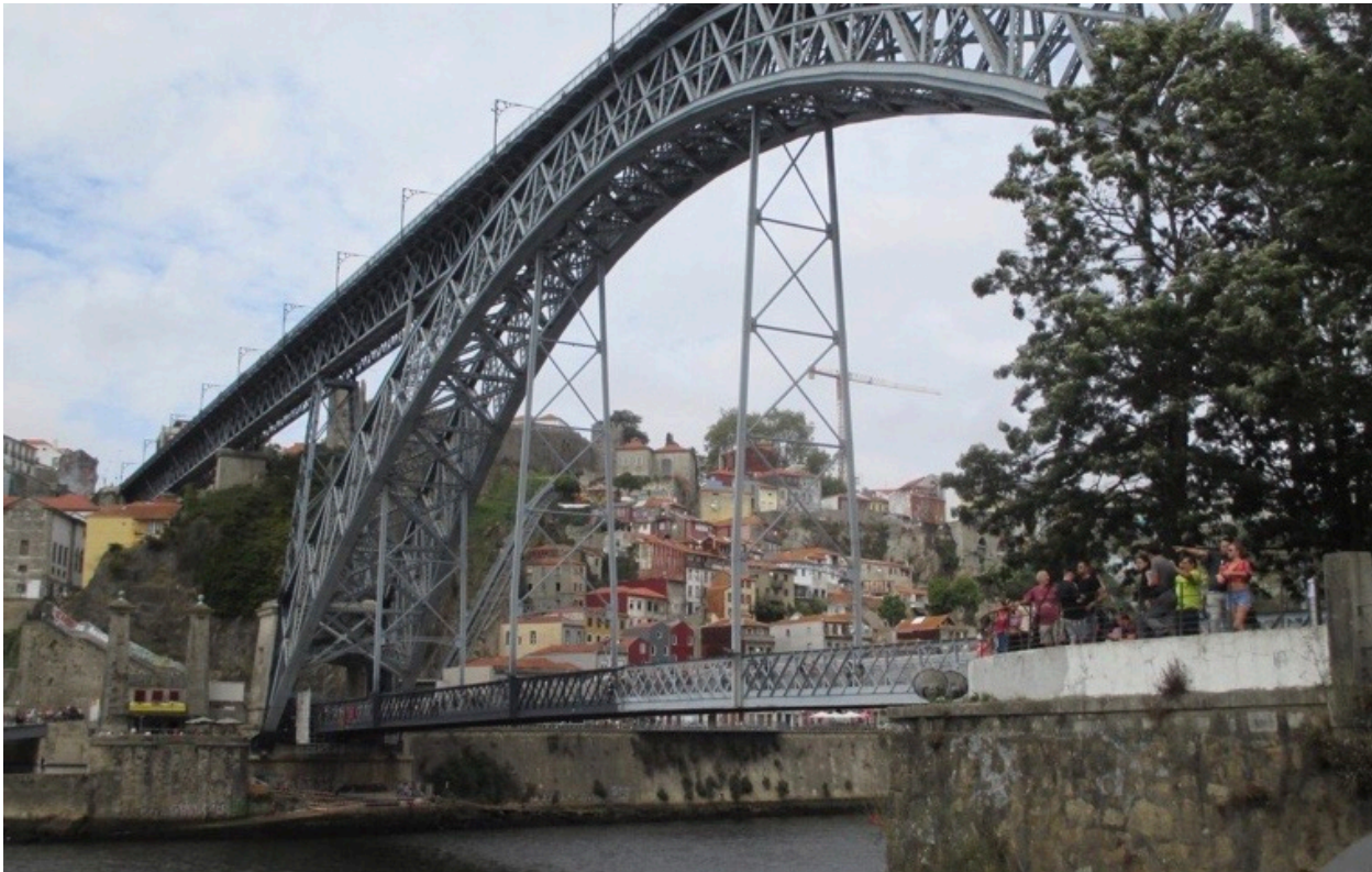
Then there's the symbol of the city, the Ponte Dom Luis I , also built by Eiffel's firm but opened 9 years after the first in 1886. It was made a double-decker to carry more traffic.
