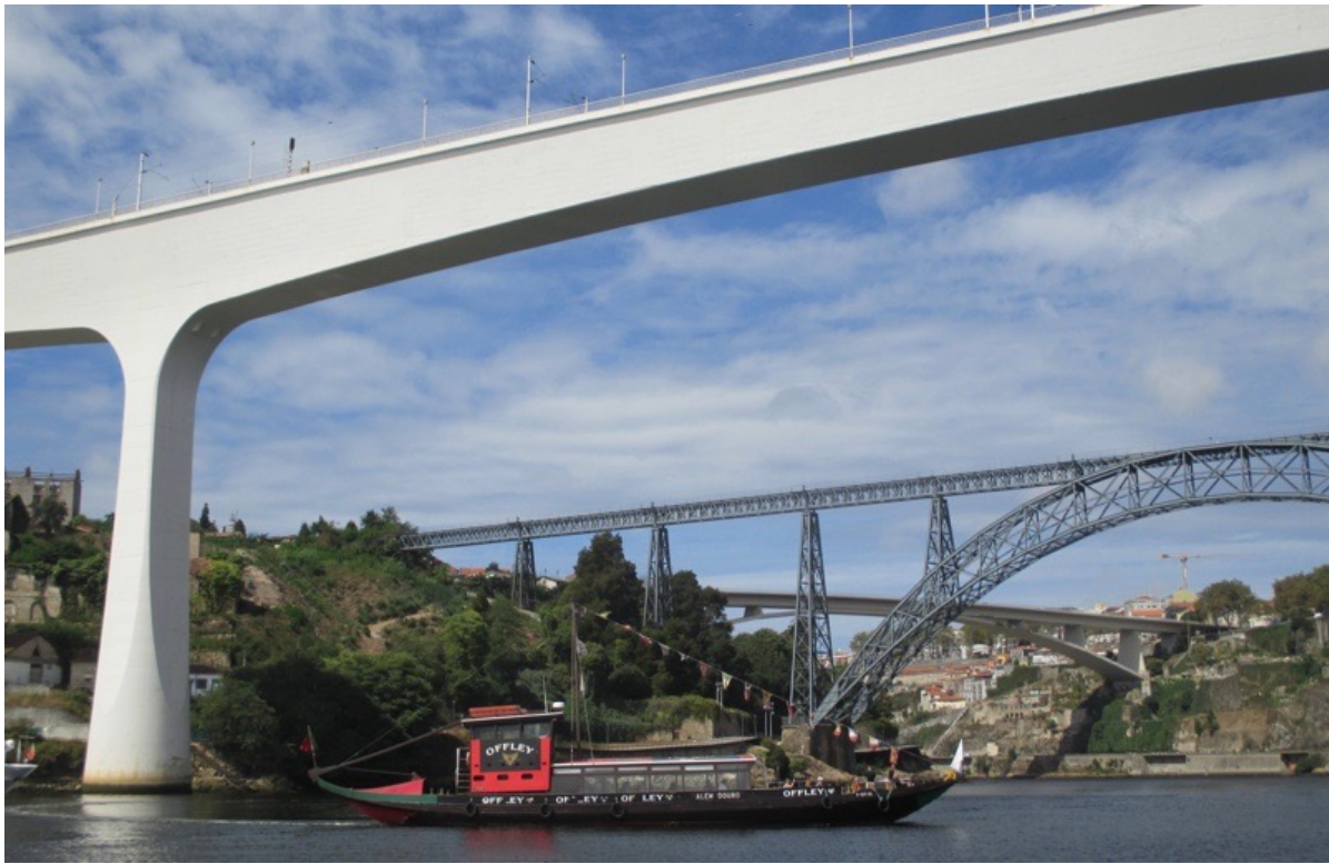
The Ponte São João bridge in front of Maria Pia took over the railroad traffic in 1991. The one behind her ( Ponte Infante ) opened in 2003 for local vehicular traffic.
