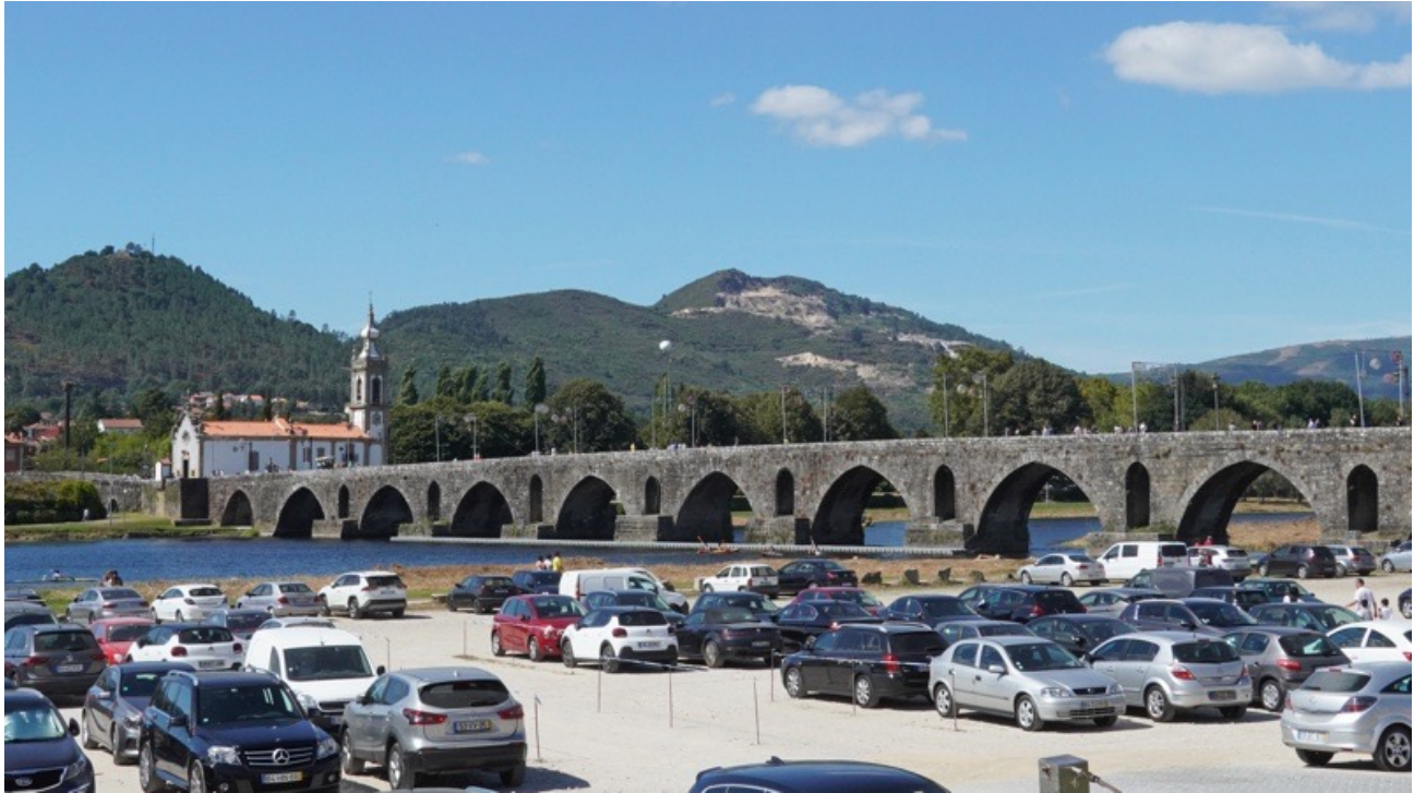
The name means “Bridge of the Lima (River)”, and here it is! This one, built in the 14th Century, mirrors the design of the original one built in the 1st Century by the Roman Empire.
