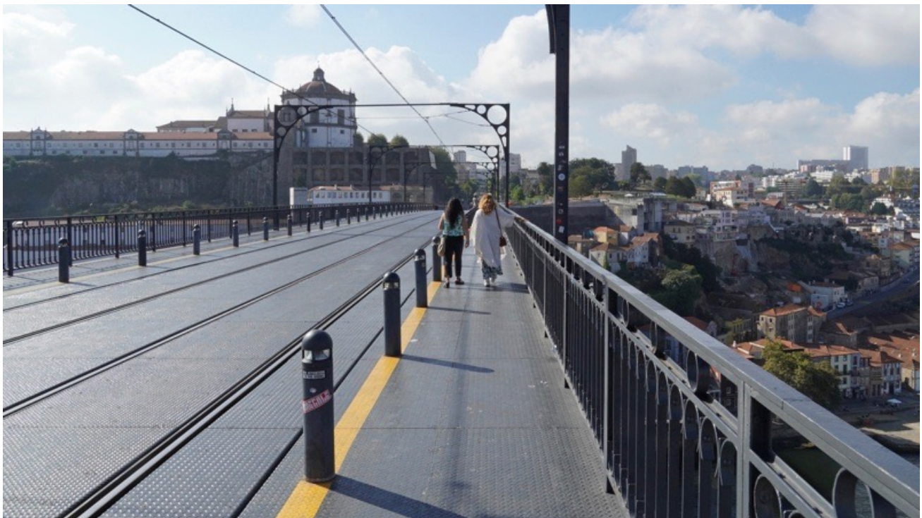
This bridge is only used by the Metro trams and pedestrians, so there's no other traffic.
