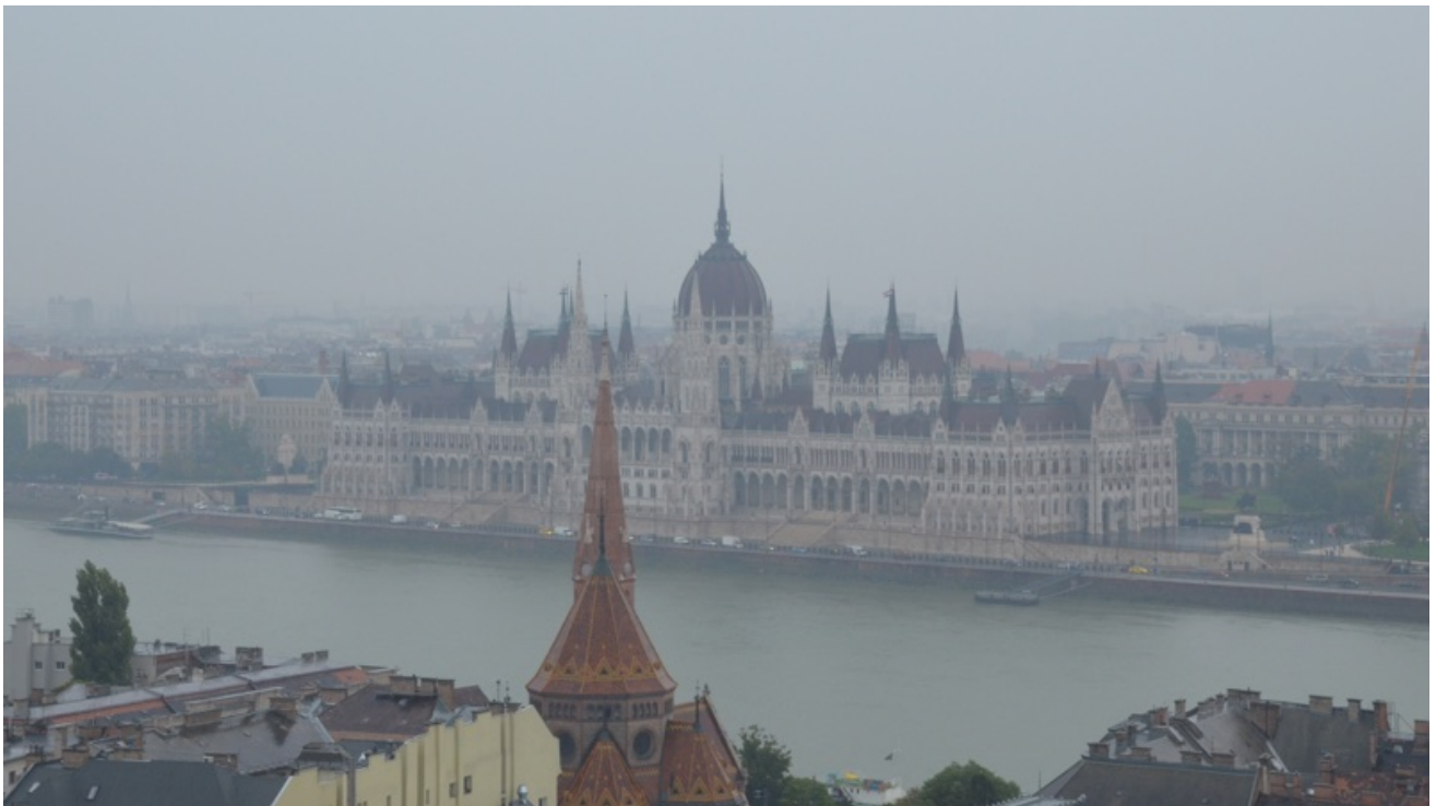
Completed in 1904, it was a statement of the wealth & power of the Austria-Hungary Empire.
